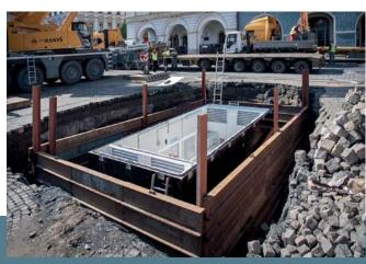
To speed up the installation, we install the electrical technology in the station at the production plant.
